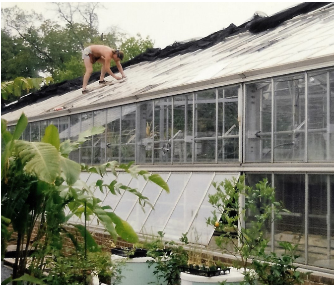
Greenhouse Hail Damage, June 1993
